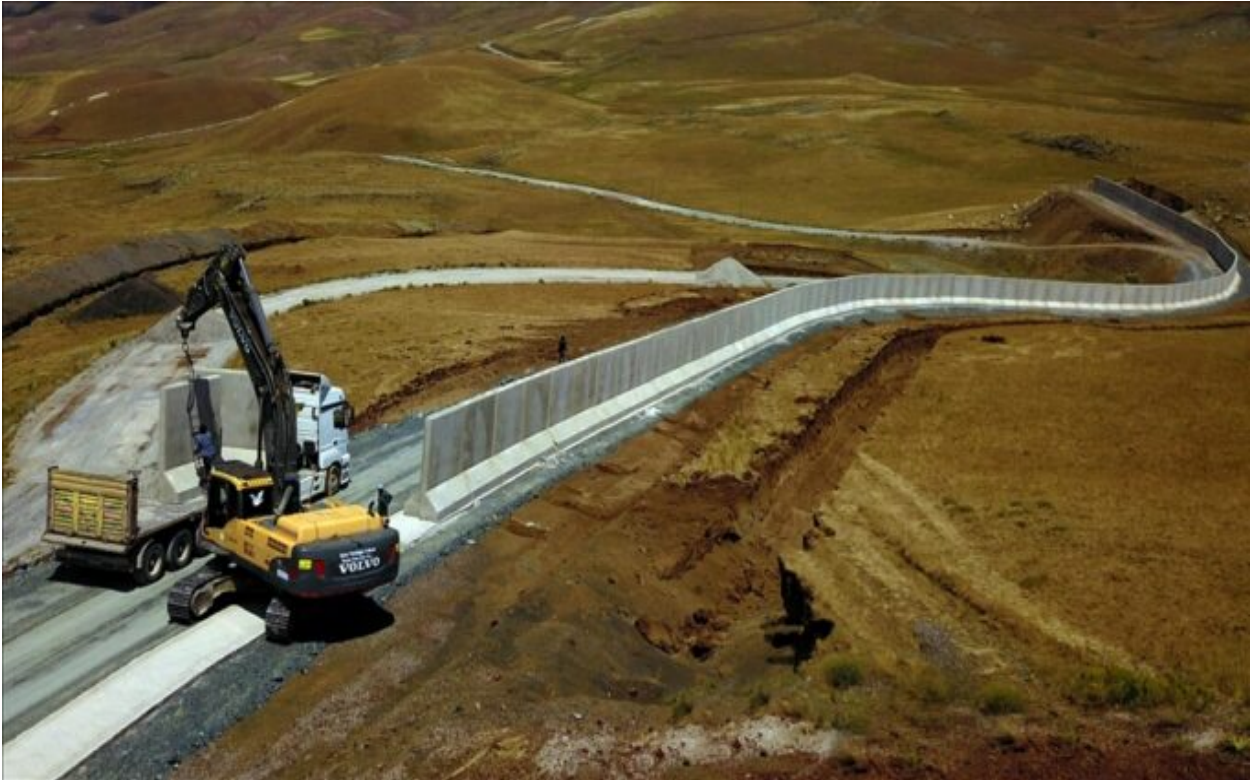
Construction of a so-called "security wall" along the Turkish-Iranian border
